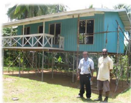
One of four houses erected in Ieran village
