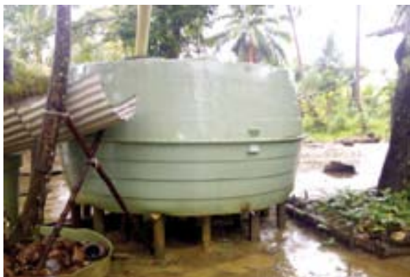
Implementation of the Middle and South Fly Water Catchment Project will see existing tanks repaired and new tanks installed in all South Fly delta villages
