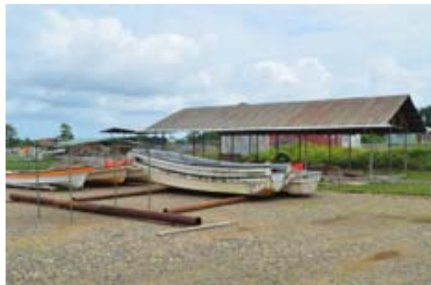
Resheeting at the OTDF Trust Yard site, Kiunga
